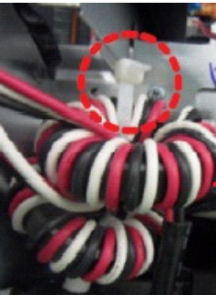
► Fix Comp Wire-Core to Bracket Beam Control Box using large size Cable Tie(350mm).
