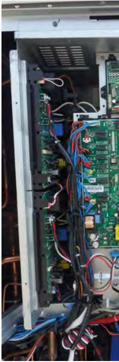
► Comp Wire fix by Holder Wire.
